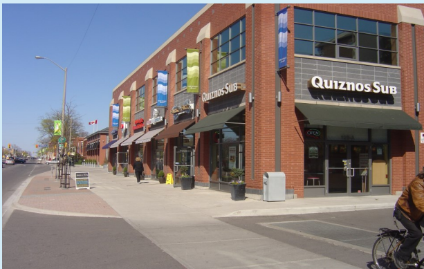
Figure B76 — Image of the Mainstreet Corridor Precinct
