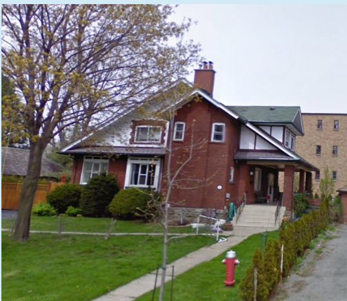
Figure C47 — 5 Oakwood Avenue North
