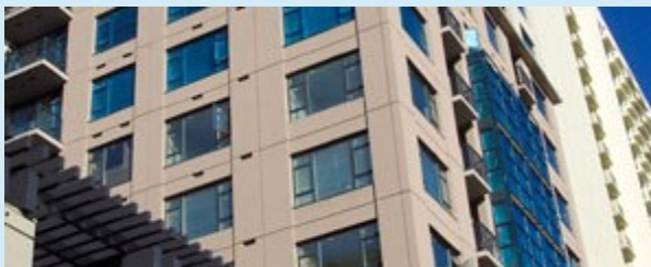
Figure B106 — EIFS Panels for more than 20% of the building material and should not be placed within the first 2 storey's
