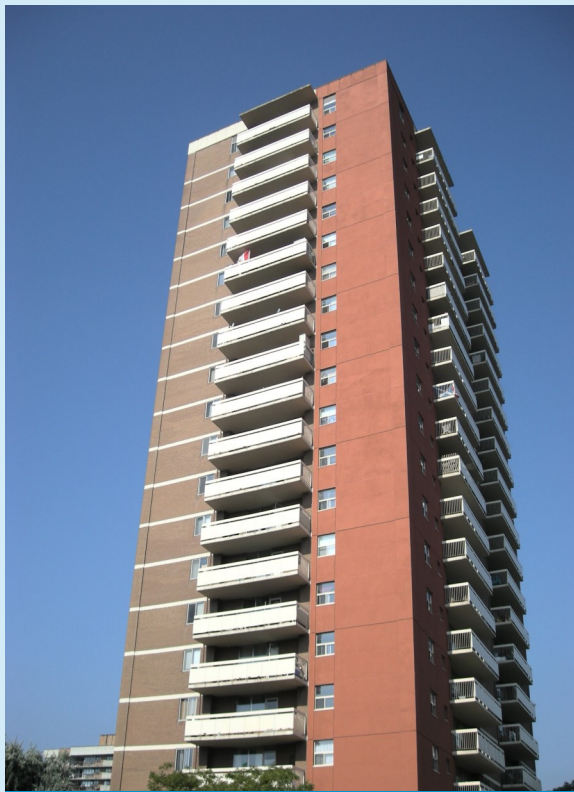
Figure B41 — Existing building in the Central Residential Precinct. Floor plate of 683 m 2
