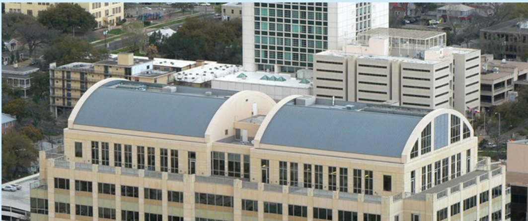
Figure B97 — Example of roof top mechanical that has been integrated and designed into the building
